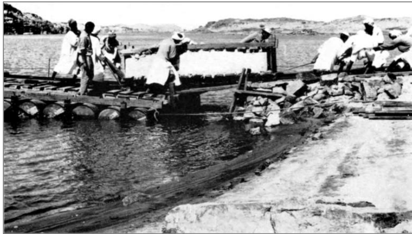
Fig. 24. Semna East: off-loading one of the 4-ton roof blocks from the pontoon (Hinkel, 1965: 104).
