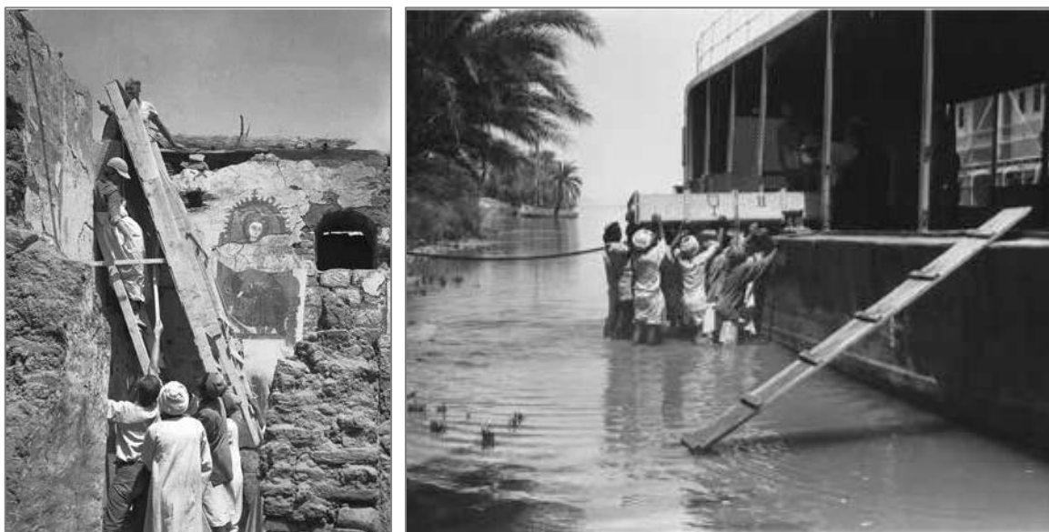
Fig. 29. Restoration work in Faras. Transportation of packed plates over the Nile to Wadi Halfa, 1964 (Jakobielski and Martens-Czarnecka, 2017: 21).
