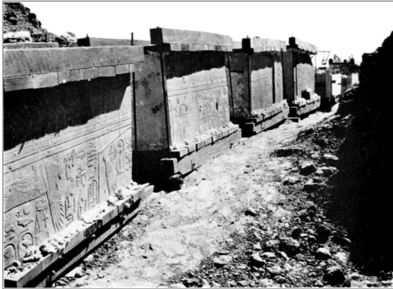
Fig. 23. Semna West: packed sandstone blocks, the sides not yet covered, waiting on the plank causeway leading to the pontoon (Hinkel, 1965: 104).
