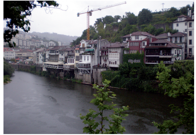
Fig. 4. Floods of level II affect the buildings cellars on the left bank.
