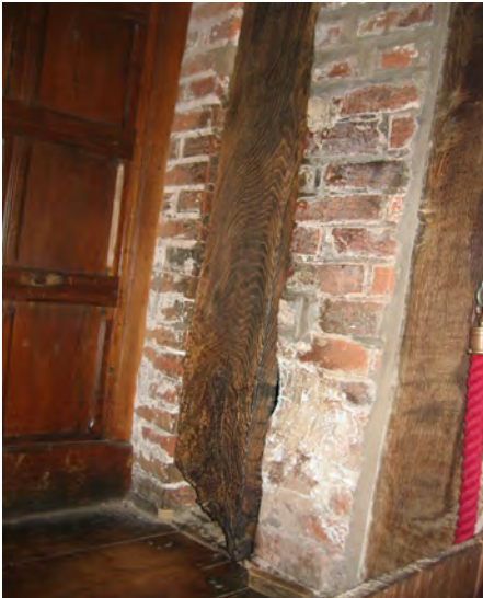
The moving beam, when closed, masked the hiding room behind the wall.
