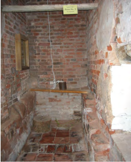
A type of priest-hide arranged in a chimney. One or two priests were seated on the beam and driven up to a special hole located on the higher floor while a fire ignited downstairs masked the real purpose of the chimney. Phot. W. Lipoński.
